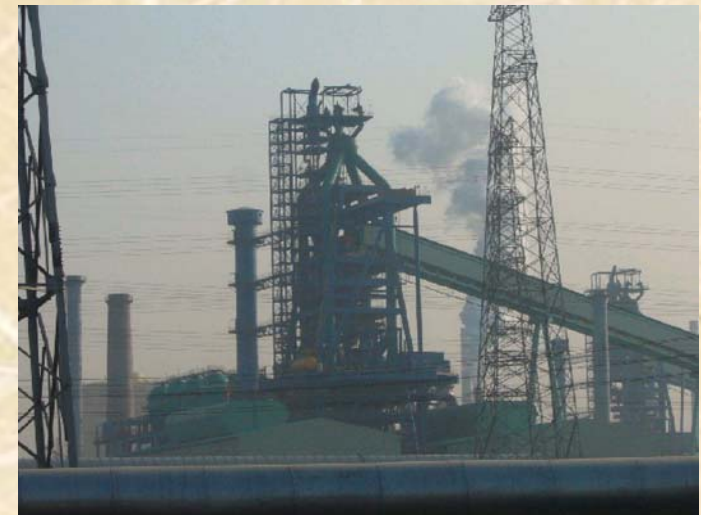
BF of new steelworks of Maanshan Steel
